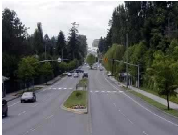
Figure 19. Use of a refuge island at a trail crossing, www.pedbikeimages.org/ - Dan Burden
