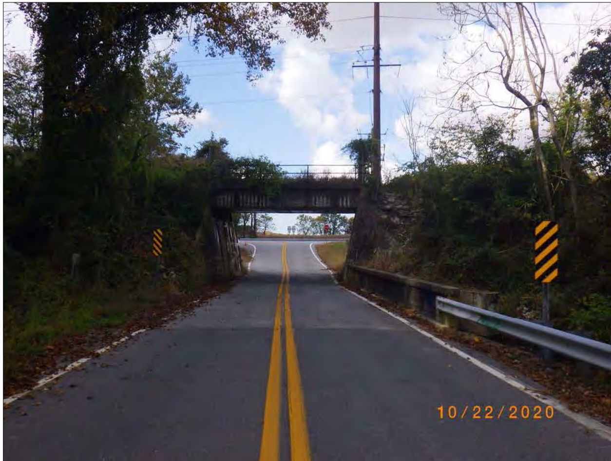
Image 18. Bridge over Tappers Corner Road, East Elevation. Credit: PrimeAE.
